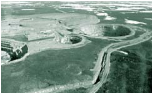
Panda Diversion Channel (in front) Koala Pit, Koala North Pit and Panda Pit (Panda/Koala waste rock pile behind) AGENCY
