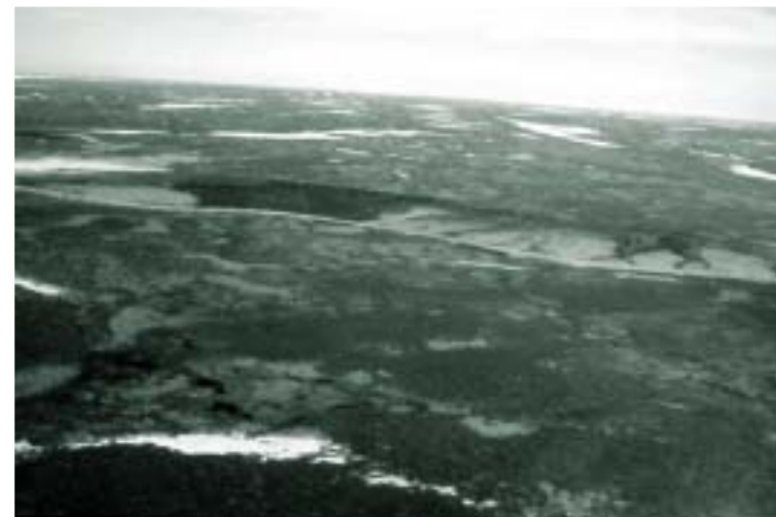
Cell B of the Long lake containment facility AGENCY
