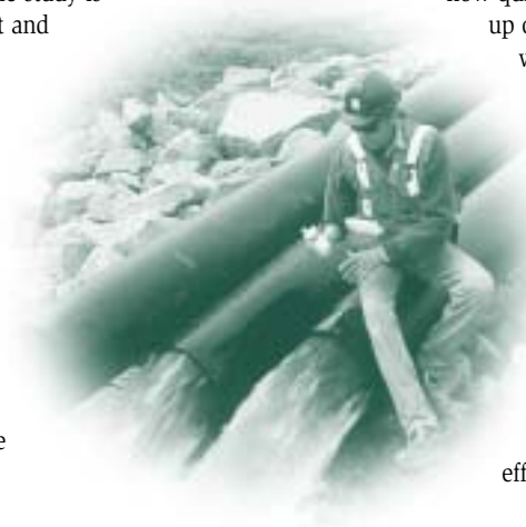
Water discharge from cell E of the Long Lake containment facility JIRI HERMANN/BHP BILLITON DIAMONDS INC.
