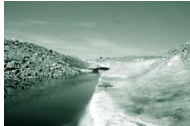
Panda Diversion Channel (spring runoff) AGENCY
