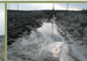
Panda Diversion Channel
